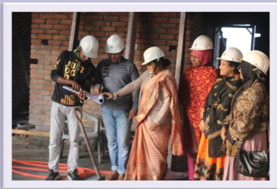
Ongoing monitoring of the 'Jibon Mela' Nursing Academic Building construction
