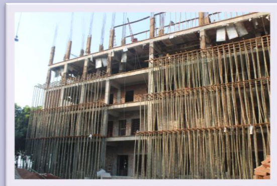
Outer view of the under construction 'Jibon Mela' Nursing Academic Building
